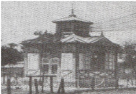
Fig. 10 Xin Gongyuan power distribution station
