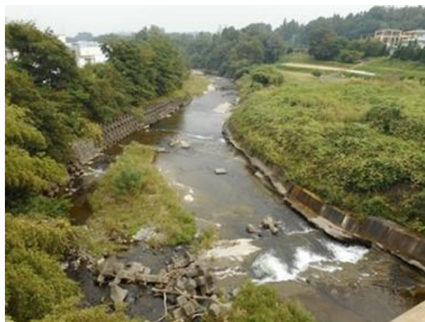
Fig. 1 Erosion of soft rocks at the bottom of the Usui River
